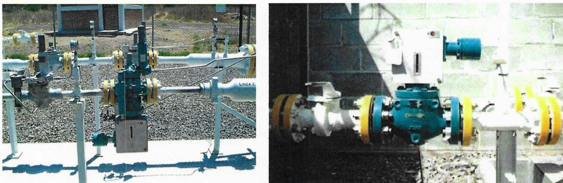
**Figura II-26: Válvula Slam Shut**
